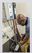
Another ongoing initiative is the introduction of stabilized aqueous ozone (SAO) cleaning technology in the Environmental Services Department of PMC. The SAO system adds oxygen to tap water to create an effective cleaning and sanitizing solution without harmful chemicals.
